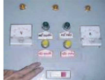
Labels for controls (Vietnam)
